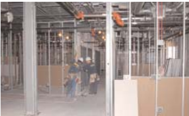
Workers begin drywalling in the second floor College of Business area.
